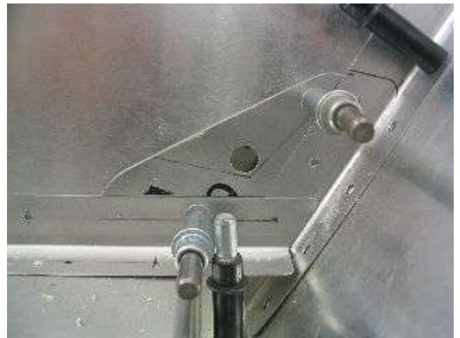
Photo 13 Shim for 6B18-3 Attachment Doubler Plate
