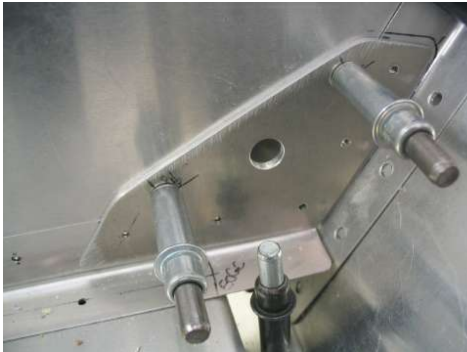
Photo 7 Installed Doubler and Shim for the inboard harness attachment
